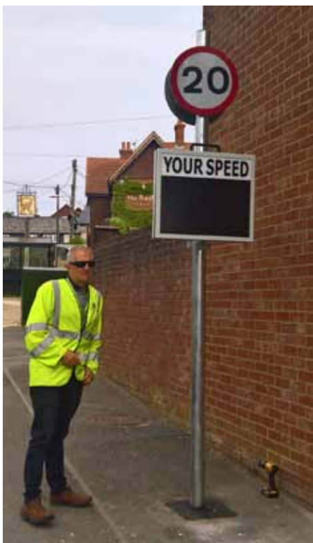
Photo of the new Speed Indicator Device (SID) being installed today on the High Street it has been sent separately. It does not record – it tells drivers how fast they are going. It will be deployed at various locations around the village.
