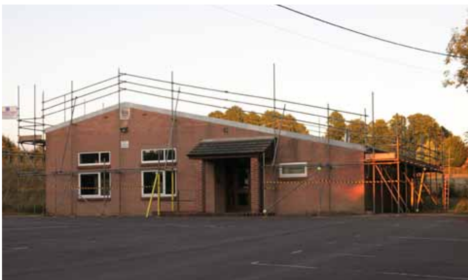
Scaffolding up on Sixpenny Handley Village Hall
